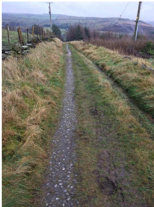
Photograph 3- Route looking towards Huddersfield Road. Metalled surface clearly visible as are horse hoof prints. Path width 12-18 feet
