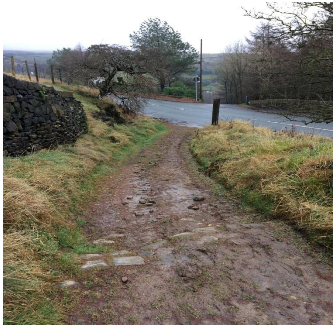
Photograph 4. Looking towards Huddersfield Road, metalling clearly visible.
