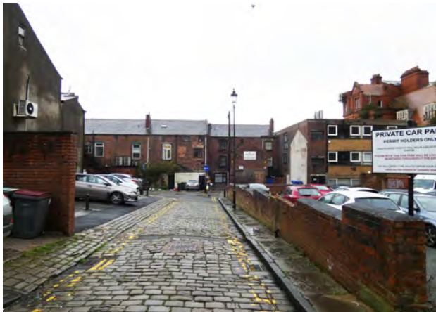
Plate 7.1 Cobbled roadway to Harrison Street
