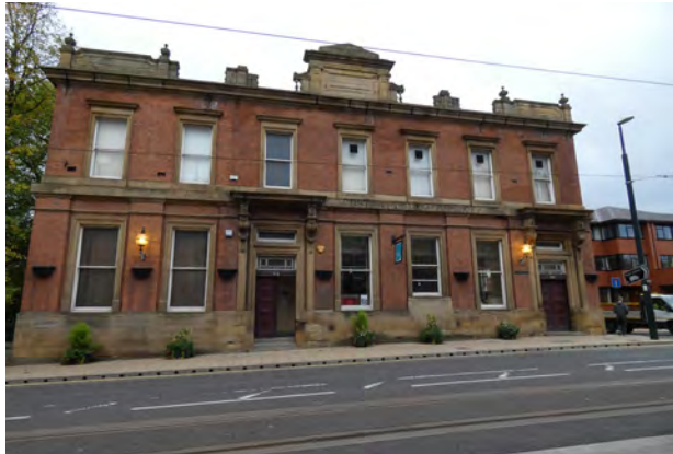
Plate 5.45 Former Post Office
