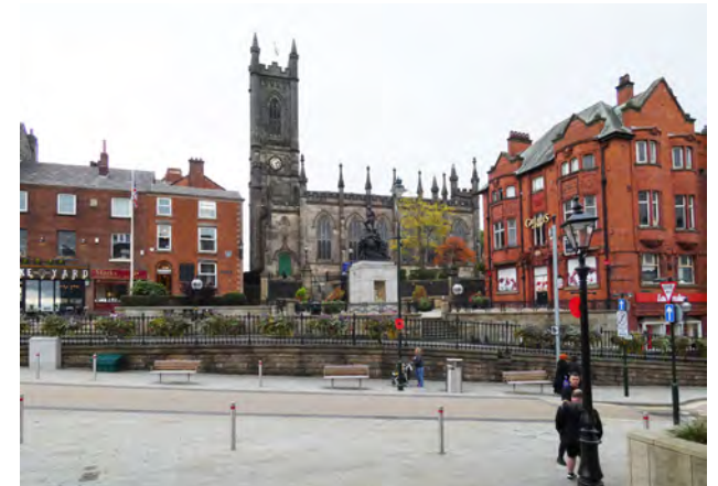
Plate 5.2 The Church of St Mary and St Peter crowning the centre of the conservation area
