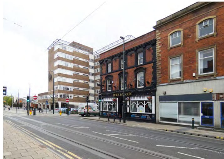
Plate 3.8 Diverse range of buildings along Union Street to west
