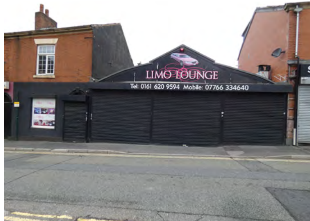
Plate 9.28 Unsightly infill within terrace group on Waterloo Street
