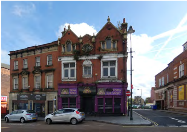
Plate 8.5 Poor condition typical of many buildings within the conservation area
