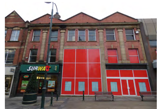
Plate 9.16 Poor signage and shopfronts within proposed extension causing harm to overall appearance of building which makes a positive contribution to the conservation area
