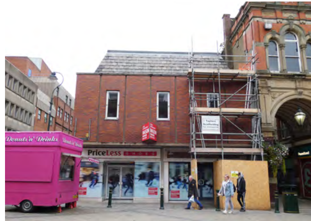
Plate 8.1 1-3 High Street detracting from the composition, scale and detailing of the Hilton Arcade block
