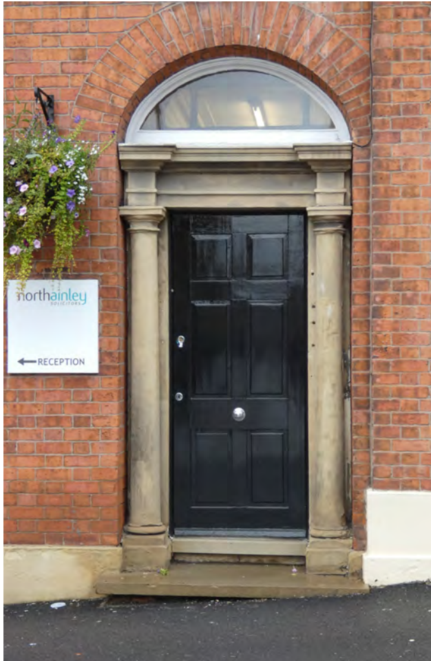
Plate 5.65 Stone doorcase to vernacular brick building on Clegg Street
