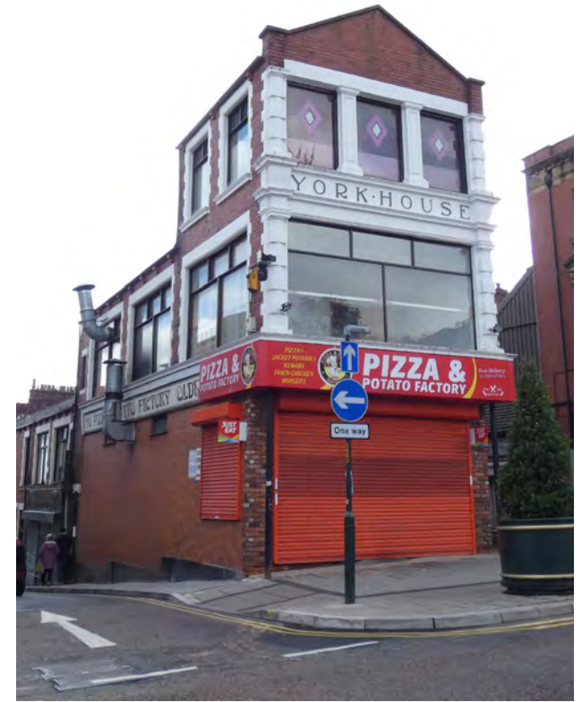
Plate 8.7 32 Yorkshire Street with poor shopfront and signage, roller shutters and unsightly flues
