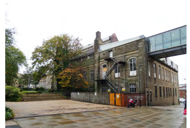
Plate 9.29 Pedestrianised public realm to south side of Cultural Quarter
