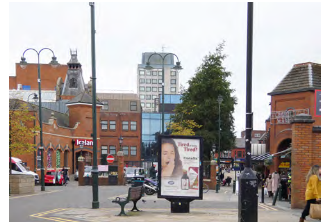
Plate 6.7 Civic centre tower sat at the opposite end of the town centre from the Church of St Mary and St Peter spire
