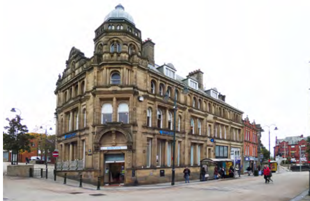
Plate 5.13 Grade II-listed Barclays Bank on the corner with Church Terrace and the Greaves Arms positioned behind
