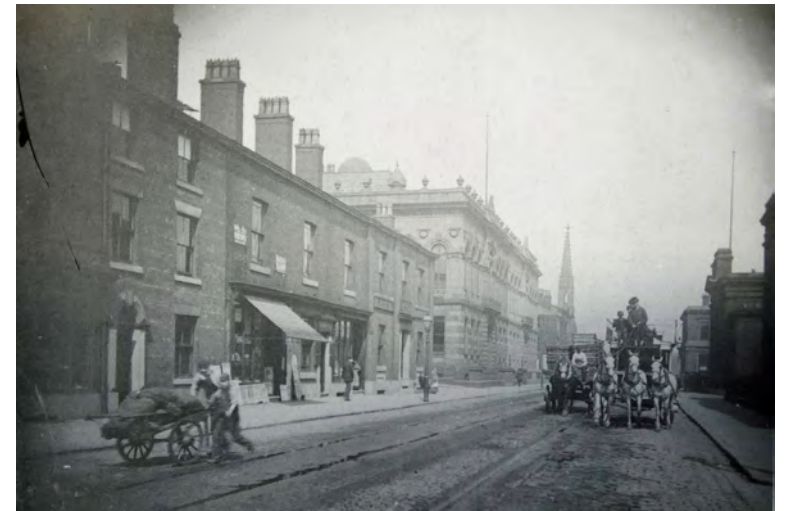
Plate 4.13 Union Street looking east, nos. 87-93 on left, c. 1880 (Oldham Local Studies & Archives)
