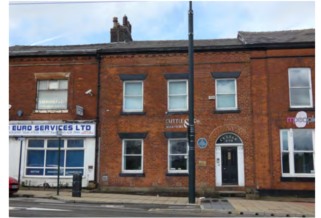
Plate 9.26 Examples of poor ground floor frontage and more sensitive solution within proposed extension on Union Street
