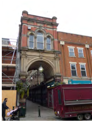
Plate 5.53 South face of Hilton Arcade
