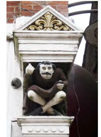
Plate 9.13 Carved capital and corbel brackets to 19 th century retail frontage on Henshaw Street
