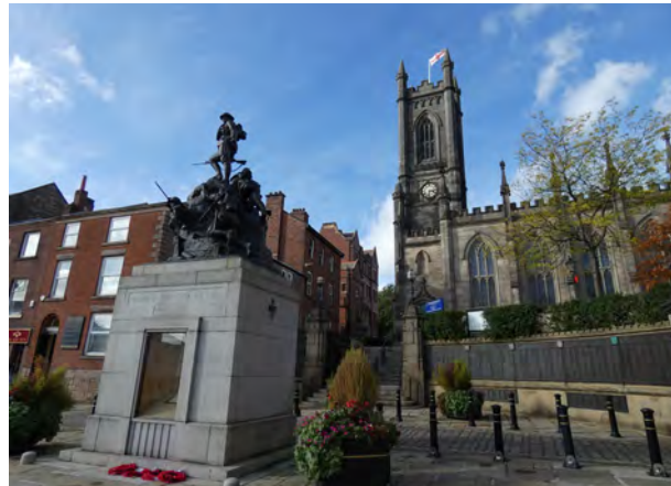
Plate 3.1 St. Mary's Church at the apex of the conservation area
