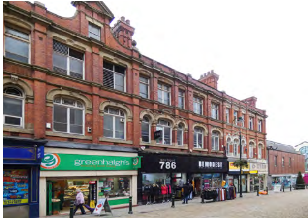
Plate 5.12 Poor retail frontage along Curzon Street at ground floor to Hilton Arcade group
